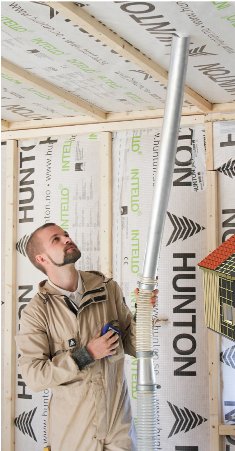
The illustration shows a wall with blow-in insulation with Nativo Wood Fibre Insulation.
